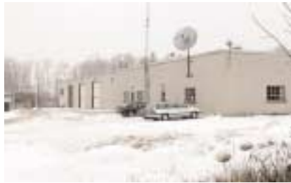
University Grounds Maintenance Facility
